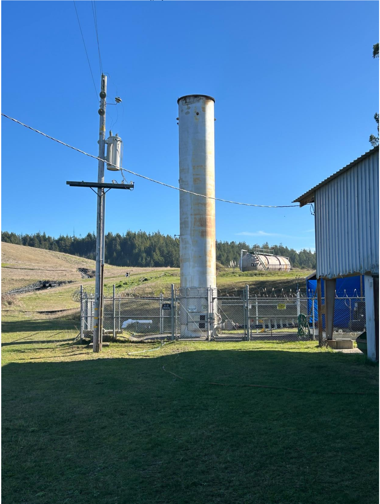
Photograph 1 – View of Flare Stack
